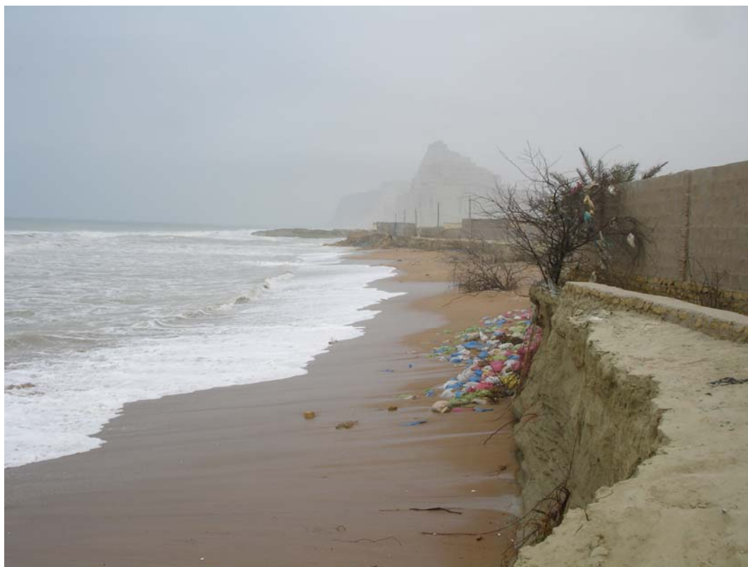
Figure 6: In Surbandar area of Gawadar, residential area is at risk from erosion. Photo credit: Ahmad Khan
